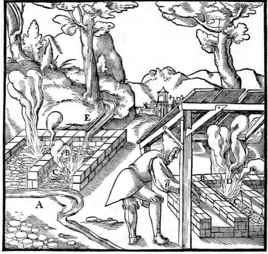
A-AREA. B-WOOD. C-ORE. D-CONE-SHAPED PILES. E-CANAL.
